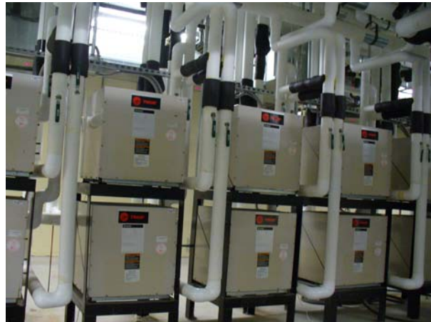
Water to Water Heat Pumps Serving AHU Coils
