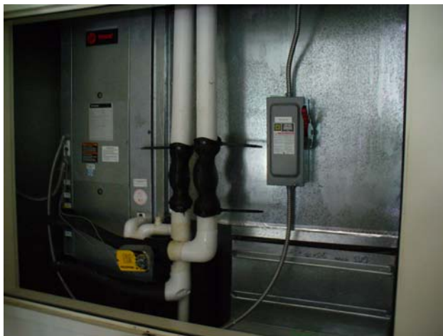
Typical Classroom Water to Air Heat Pump
